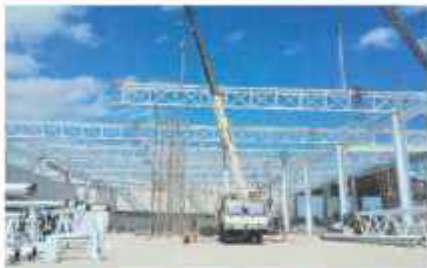
Terminal Main Building Syamsudin Noor Airport - South Kalimantan
