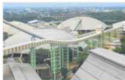
Conveyor Indocement Plant - West Java
