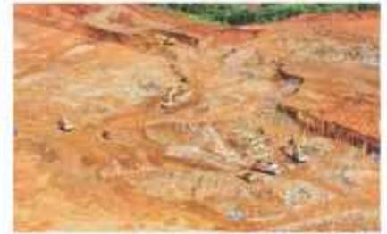
Land Development Smelter Kolaka Project - South East Sulawesi
