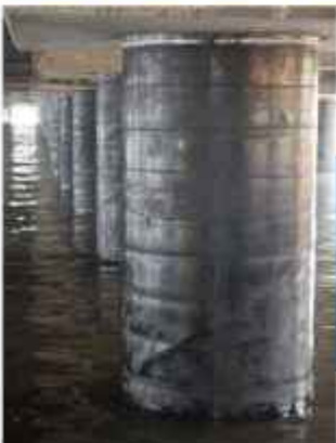
HDPE JACKETING OR COMPOSITE WRAPPING FOR SPLASH ZONE PROTECTION
