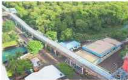
Mobile Conveyor PLTU Suralaya - Banten
