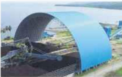
Coal Sheds PLTU 2x50 MW - Central Sulawesi
