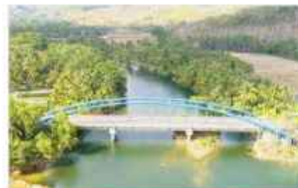
Soge Pacitan Bridge - East Java
