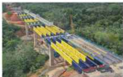
Padang Pekanbaru Toll Road Project - West Sumatra
