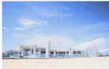
Terminal Main Building Sultan Hasanuddin International Airport - South Sulawesi
