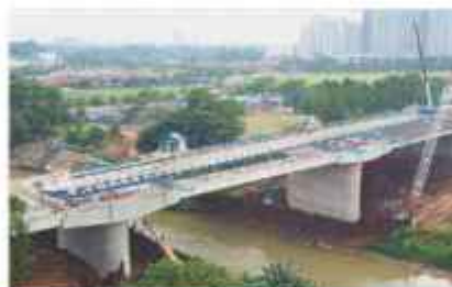
Toll Serpong Balaraja Project - Banten
