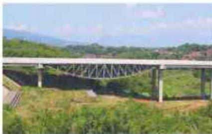
Cisumdawu Toll Road - West Java
