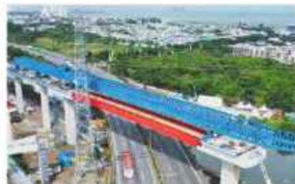
Jalan Tol Ancol Timur - Pluit (Elevated) Harbour Road II
