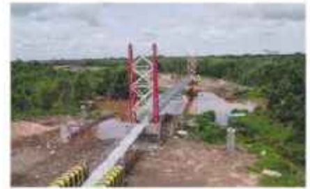
Trial Assembly - Majalengka Steel Factory
