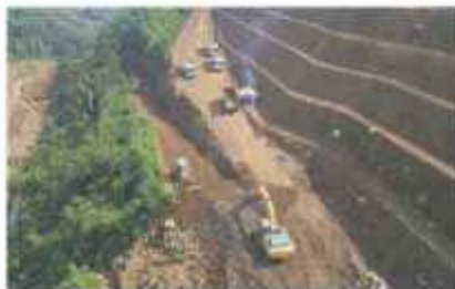
Sukamahi Dam Project - West Java
