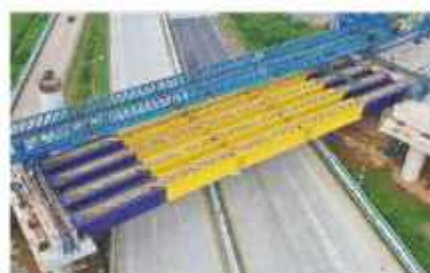
Jakarta Cikampek II Toll Road Project
