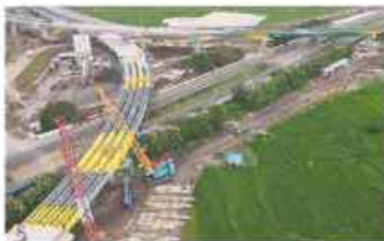
Dawuan Junction Toll Road - West Java
