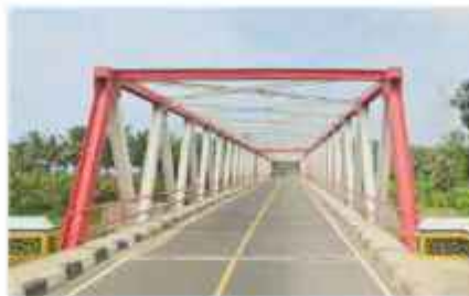
Cislih Bridge Project - Banten
