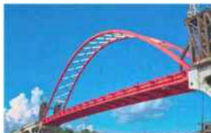
Tumbang Samba Bridge - Central Kalimantan
