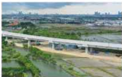
Teluk Lamong Port Access Project - East Java
