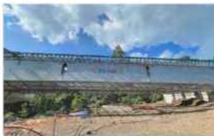
Manado Bitung Toll Road - North Sulawesi
