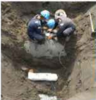
MAGNESIUM ANODE FOR UNDERGROUND PIPE LINES
