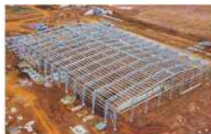
PEB 60m span structure without central support Smelter Feronike Kolaka - Southeast Sulawesi
