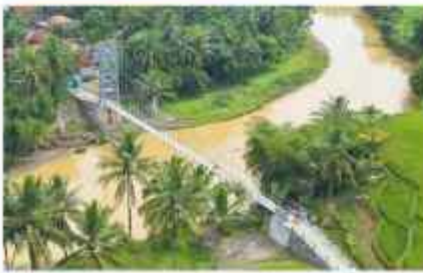
Asimetris Suspension Bridge Span 60 - Banten
